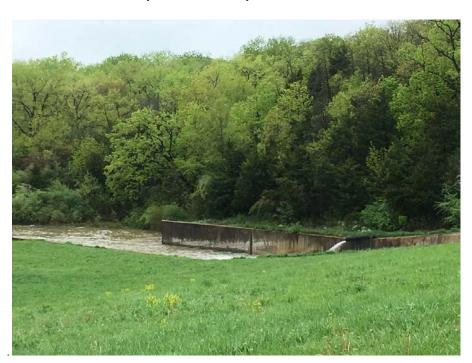
Figure 8 Seepage Bypass from the Sugar Creek Lake Dam to the Lake Spillway
